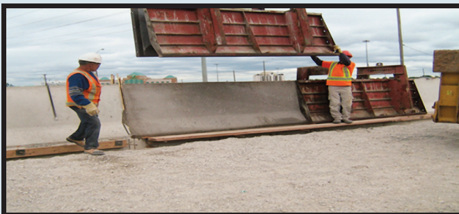
Figure 4. Bridge walls cured in less than two hours in subzero temperatures in Ontario, Canada. Credit: NanoArchitech.
